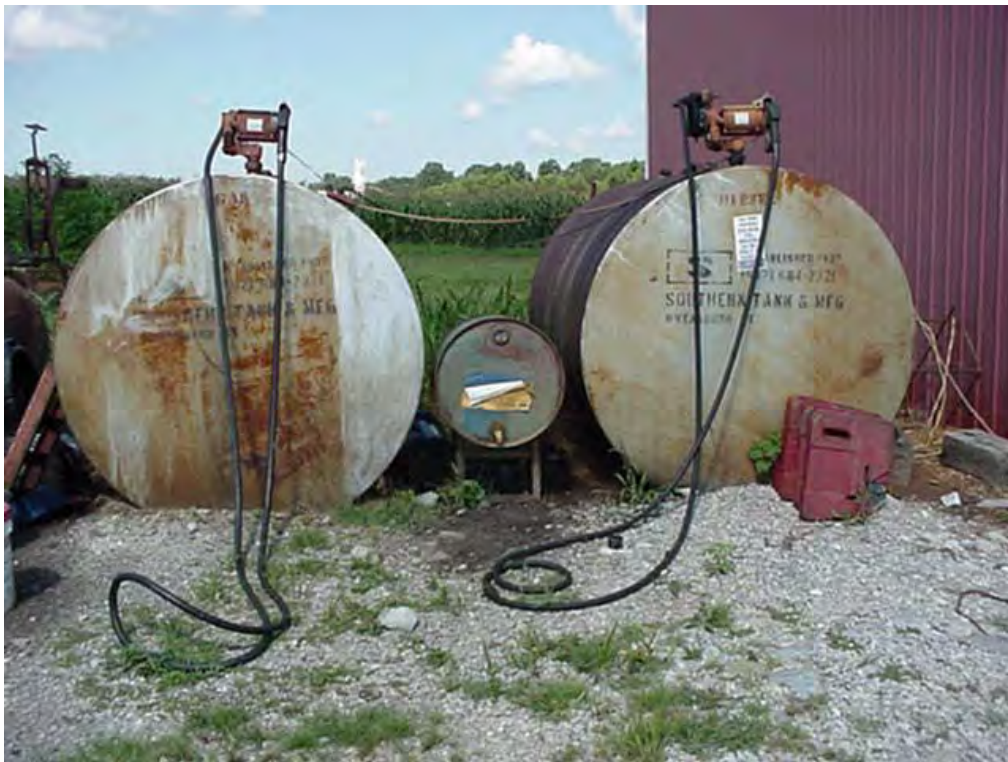
Parcel #29 – N 36° 53' 45.0", W 88° 40' 34.1" – Above Ground Diesel Storage Tanks
