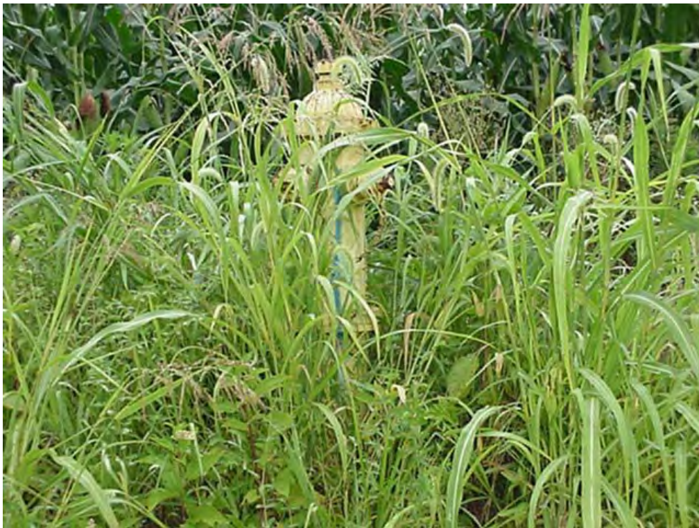
Parcel #34 - N 36° 53' 37.7", W 88° 39' 59.8" - Fire Hydrant
