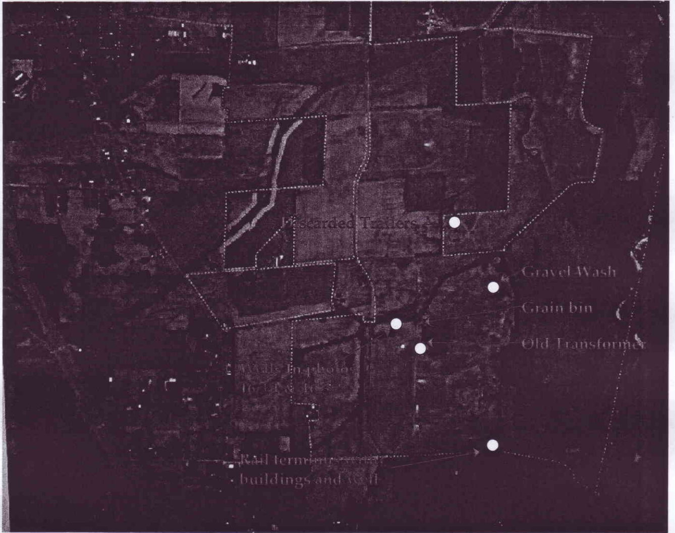
Figure 16.4.2. Aerial photo showing locations of features in text and/or photographs. North is toward the top.
