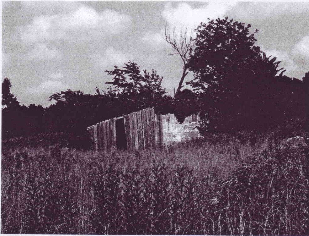
Figure 16.3.8. Building formerly used as swine pen. It consists of an addition to existing shell loading plant structure.
