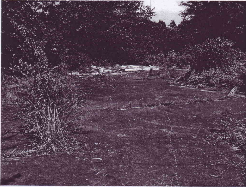
Figure 16.3.6. One of the remnant foundation of shell plant building.
