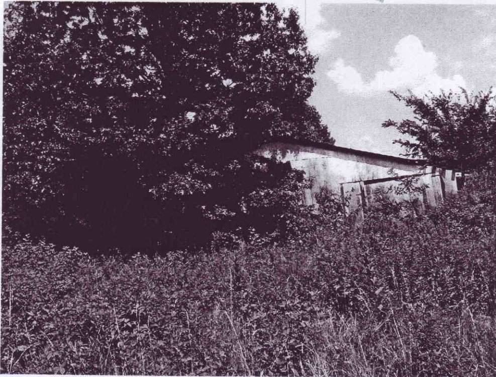
Figure 16.3.7. Building formerly used for farrowing pigs. It consists of an addition to existing shell loading plant structure.
