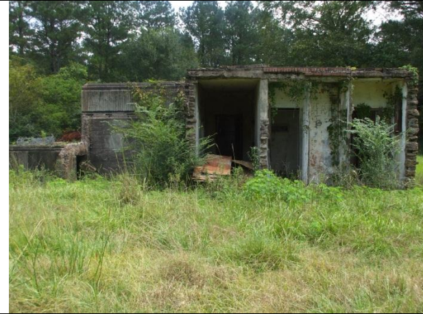
PHOTO 54 – MDAH Inventory Number 091-COL-1204 “Jail” – front (west) façade
