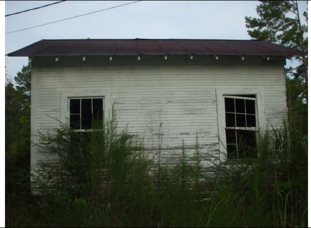
PHOTO 23 – West side of Outbuilding
