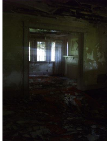
PHOTO 43 – SUPERINTENDENT'S HOME formal dining area. The floor has deteriorated and is unstable; therefore, the survey of the interior was limited due to safety concerns.
