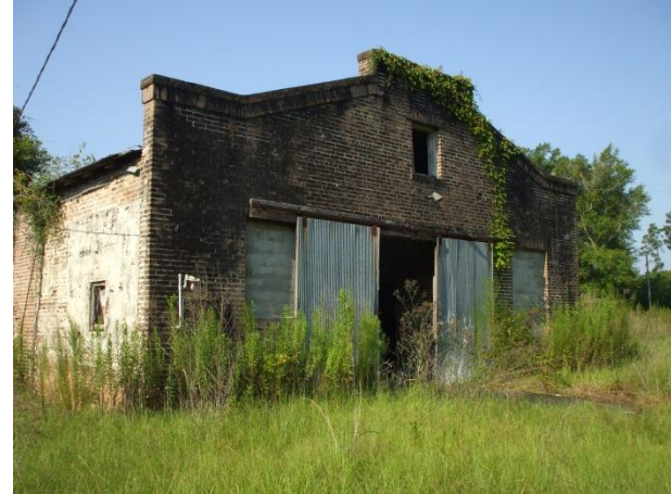
PHOTO 50 – Front façade (north side) of POWER PLANT
