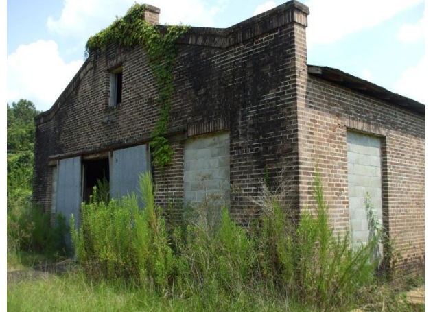
PHOTO 51 – Front façade (north side) of POWER PLANT
