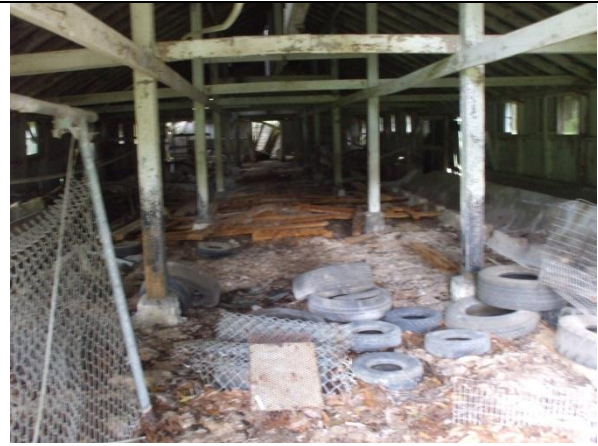
PHOTO 29 – Interior of the Dairy Barn
