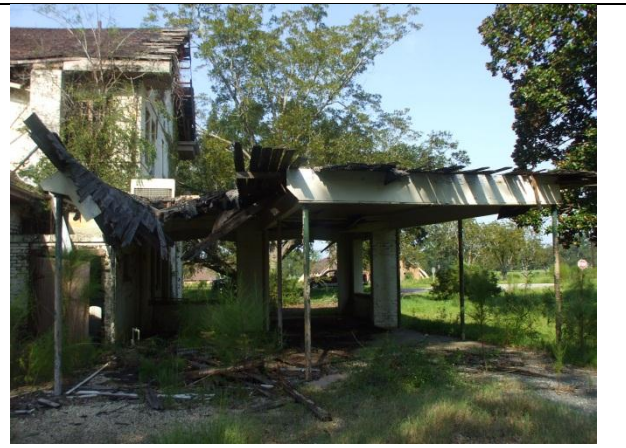
PHOTO 41 – SUPERINTENDENT'S HOME rear view of carport addition
