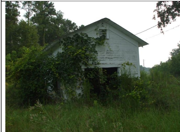
PHOTO 24 – Front (south) façade of Outbuilding
