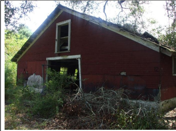
PHOTO 26 – Dairy Barn front façade (north side)
