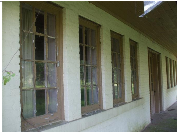
PHOTO 44 – SUPERINTENDENT'S HOME front façade windows
