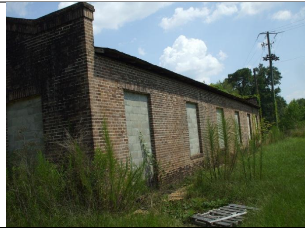
PHOTO 52 – West side of POWER PLANT
