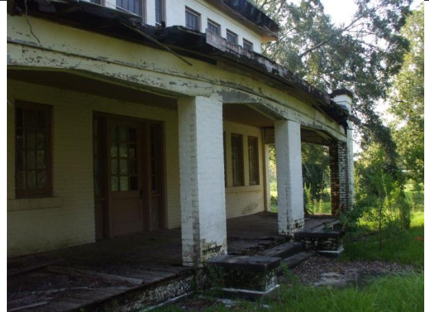
PHOTO 39 – SUPERINTENDENT'S HOME front façade
