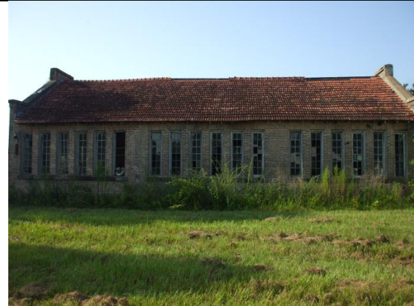
PHOTO 48 – North side of LAUNDRY BUILDING
