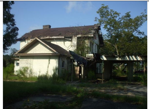
PHOTO 40 – SUPERINTENDENT'S HOME rear view
