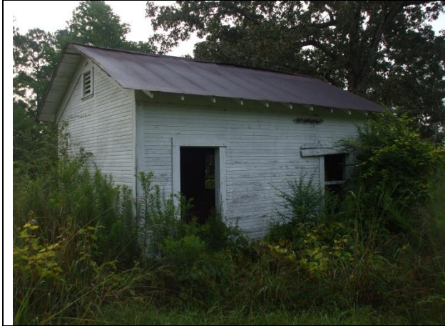
PHOTO 22 – Northwest side of Outbuilding
