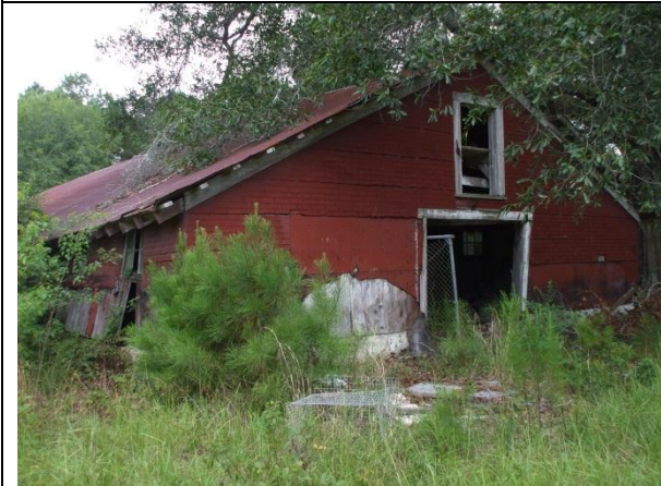
PHOTO 28 – Dairy Barn front façade (north side)
