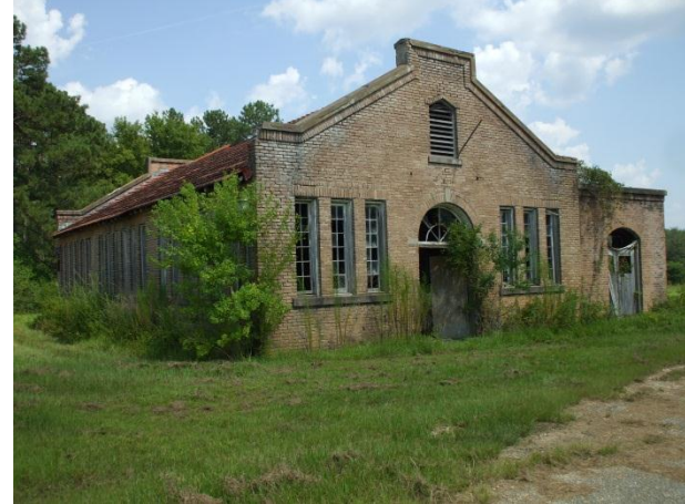
PHOTO 46 – Front façade (west side) of LAUNDRY BUILDING
