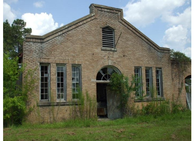
PHOTO 47 – Front façade (west side) of LAUNDRY BUILDING
