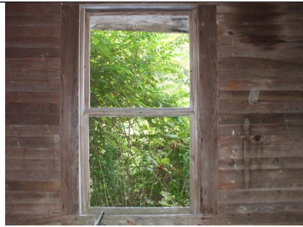
PHOTO 25 – Interior side of window of Outbuilding
