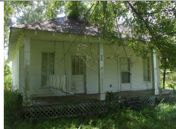
PHOTO 56 – MDAH Inventory Number 091-COL-1209 “Staff House” – front (west) façade
