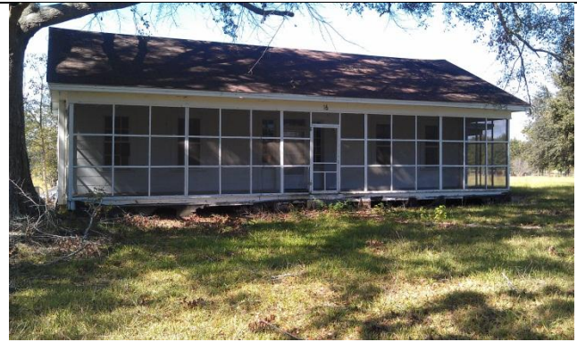
PHOTO 57 – MDAH Inventory Number 091-COL-1205 “Teacher’s House” – front façade
