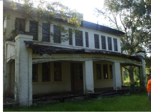
PHOTO 38 – SUPERINTENDENT'S HOME front façade
