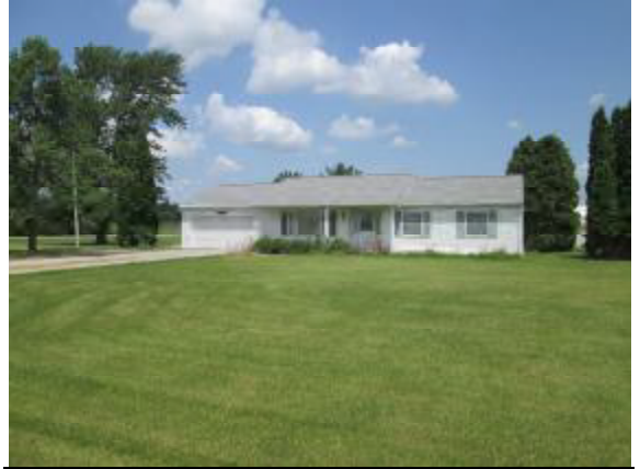
Photo #8: Viewing the vacant residence located on the southwest Site boundary.
