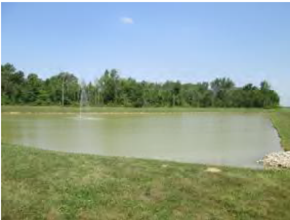
Photo #3: Viewing the northern-most retention pond.
