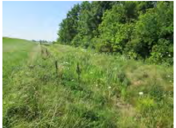
Photo #10: Viewing the drainage ditch that drains into the northern-most retention pond.
