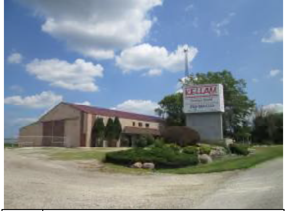
Photo #14: South adjoining commercial property.
