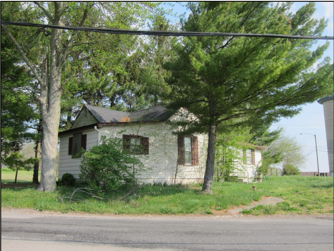
Photo 12: Facing north from Lovers Lane and showing the south and east facades of AL 4
