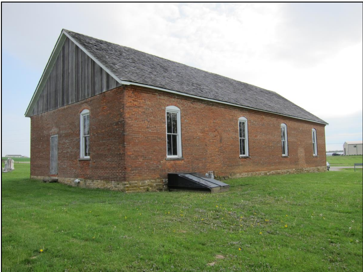
Photo 6: West and south facades of AL 2 (HIG-00223-01)
