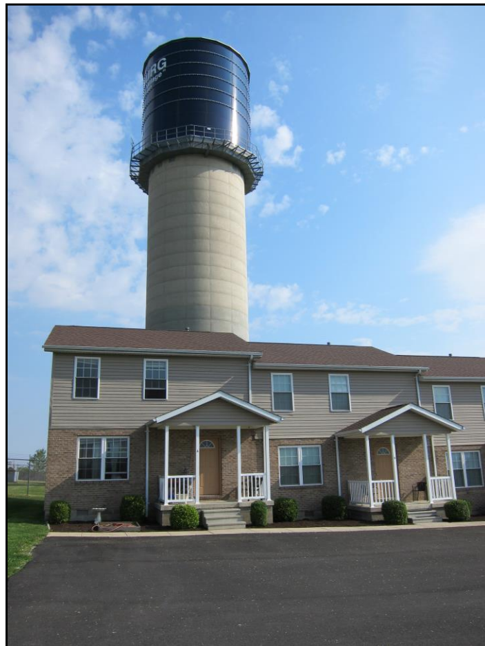
Photo 16: Facing north and showing AL 5 and AL 6
