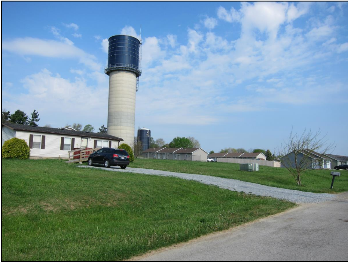
Photo 15: Facing north from Kimberly Street and showing AL 5 and AL 9
