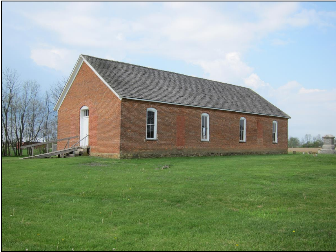
Photo 5: East and north facades of AL 2 (HIG-00223-01)
