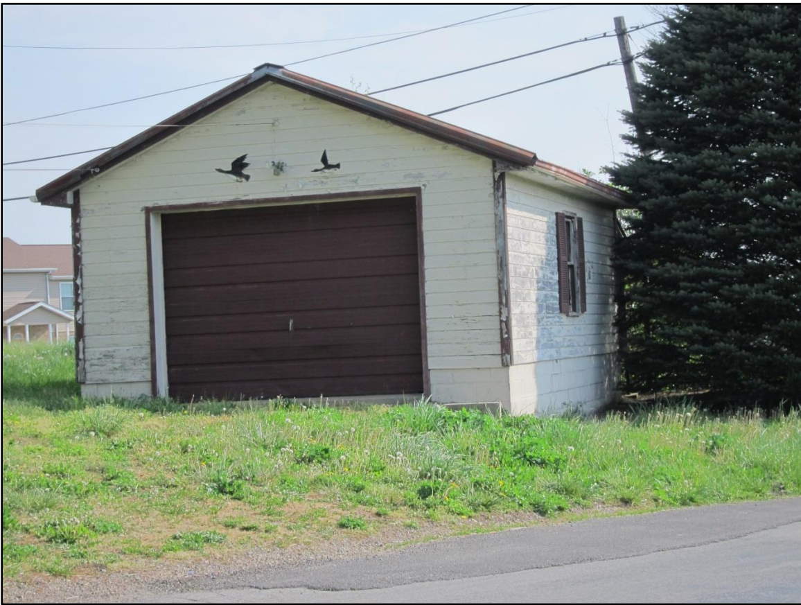
Photo 13: Facing northeast from Lovers Lane and showing the garage associated with AL 4
