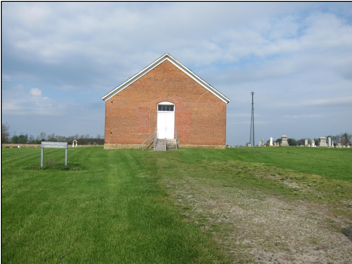
Photo 4: East facade of AL 2 (HIG-00223-01)
