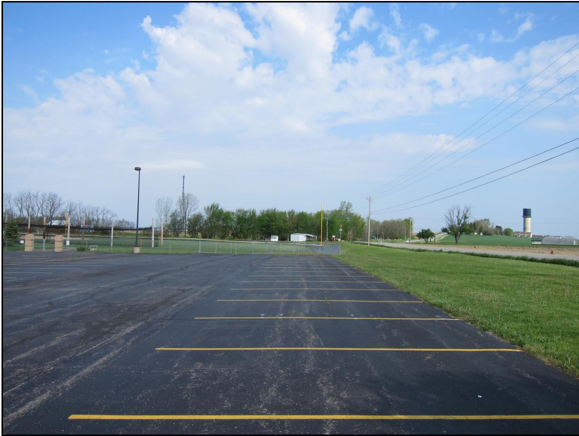
Photo 25: Facing north from AL 15, on the west side of SR 771, towards the Leesburg Industrial Park
